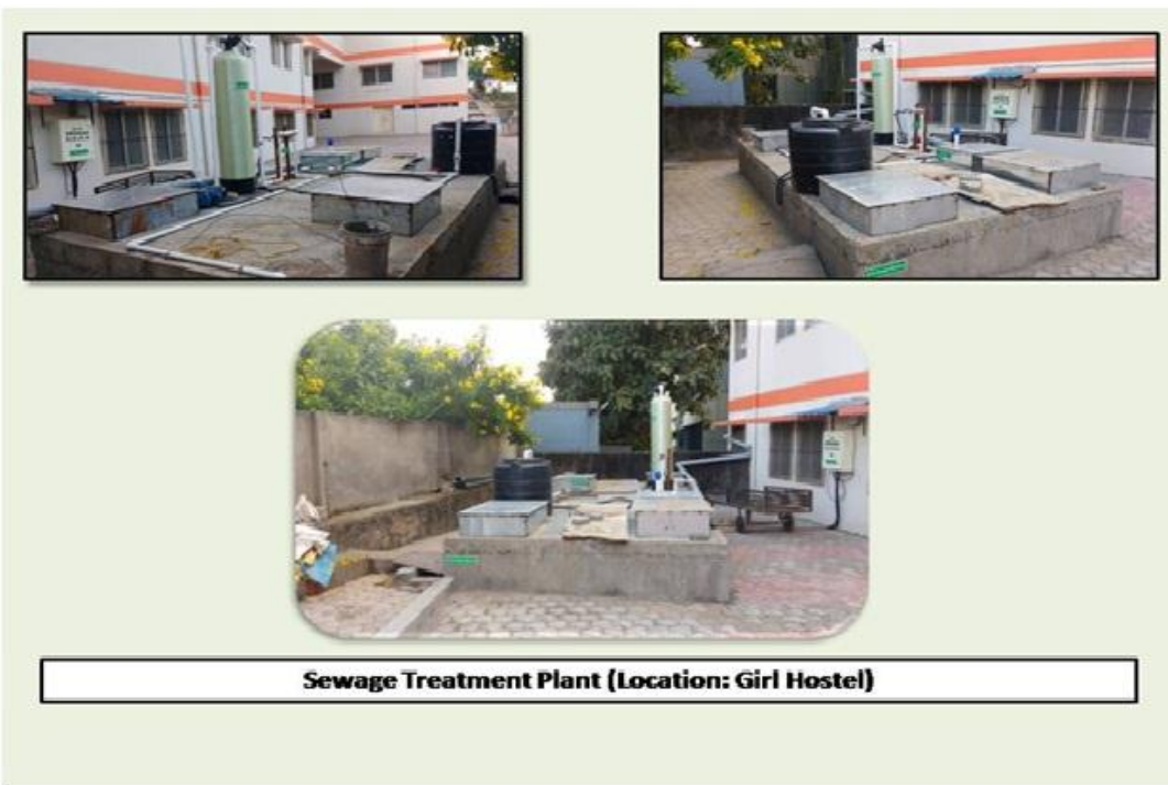
Plate No.4 : STP near Girl's hostel 25 (MLD)
